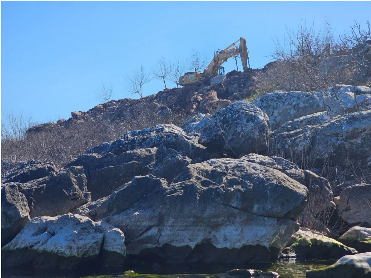
Figure 9. Construction of the new road 20-40m far from shoreline in Zogaj village.
